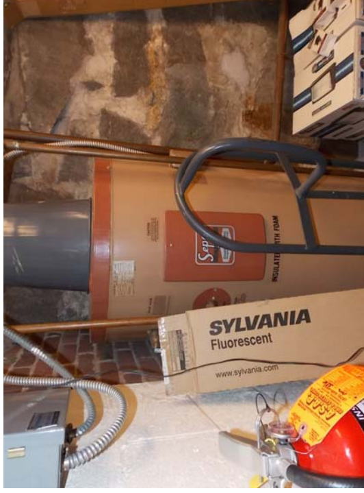
This 80-gallon electric heated DHW tank serves the entire facility.
