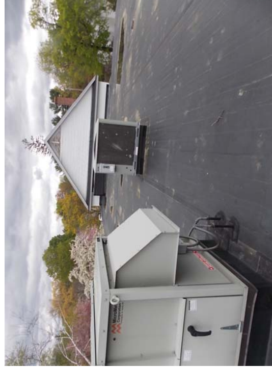
A view of the rubber membrane roofing (over the main portion of the school and several rooftop units. In the background is the original building wing.
