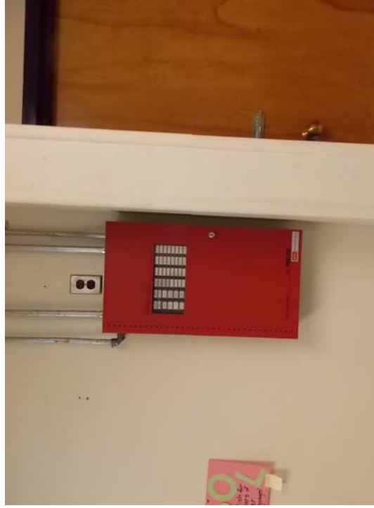
A view of the fire alarm control panel (FACP).
