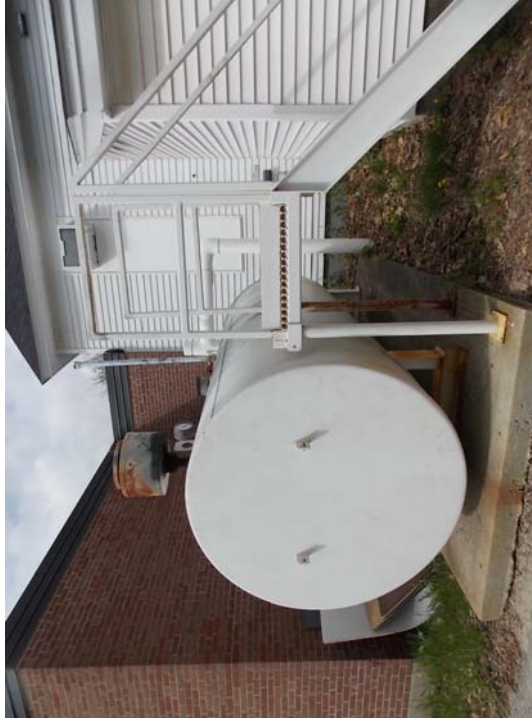
This is the above-ground double wall fuel oil storage tank.
