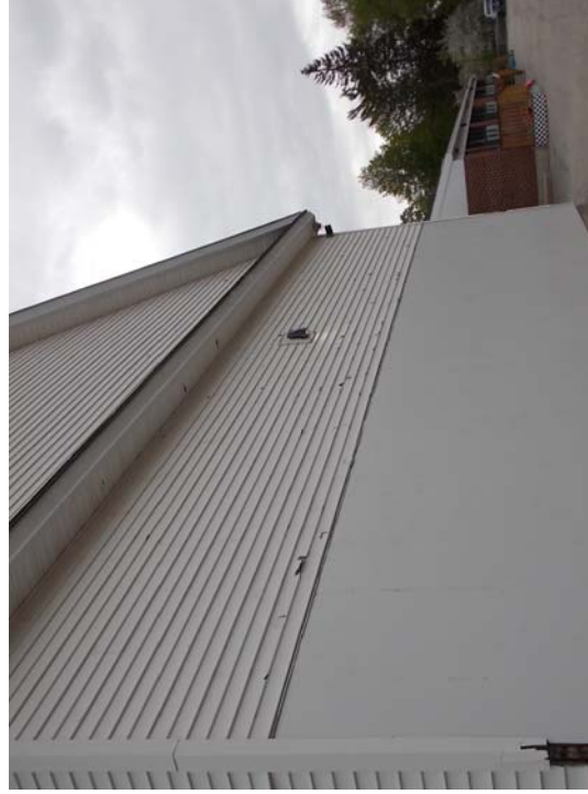
The vinyl siding on the newer building wing has areas of impact damage.
