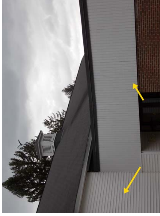
The building is clad with vinyl (left arrow), T1-11 (right arrow) and brick.
