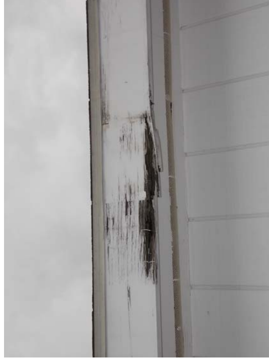
A close-up of deteriorating wood trim above the T1-11 siding.
