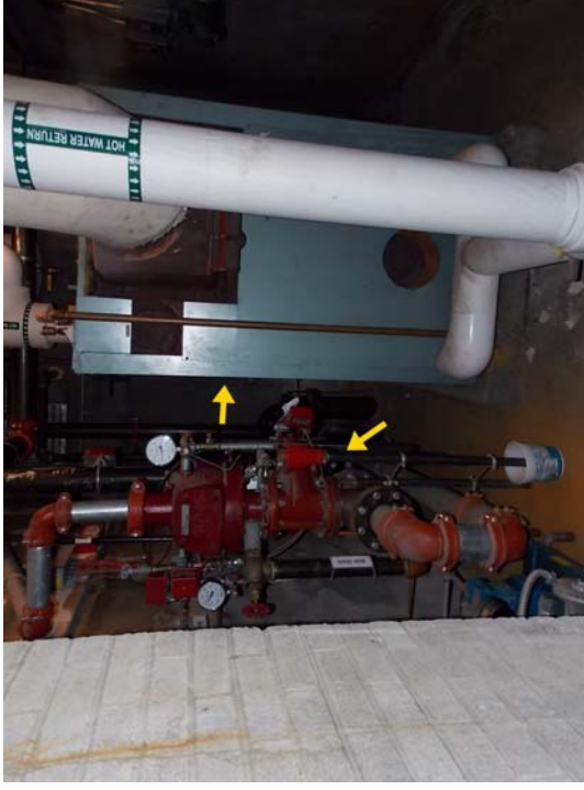
The original oil-fired boiler is on the right and the fire sprinkler connection is on the left.
