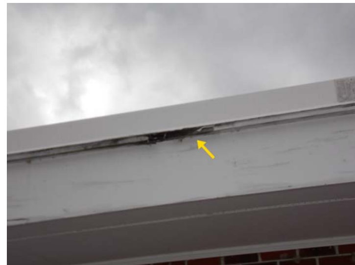
A close-up of damage at the top of a fascia board (wood trim near the roof line of the main building).
