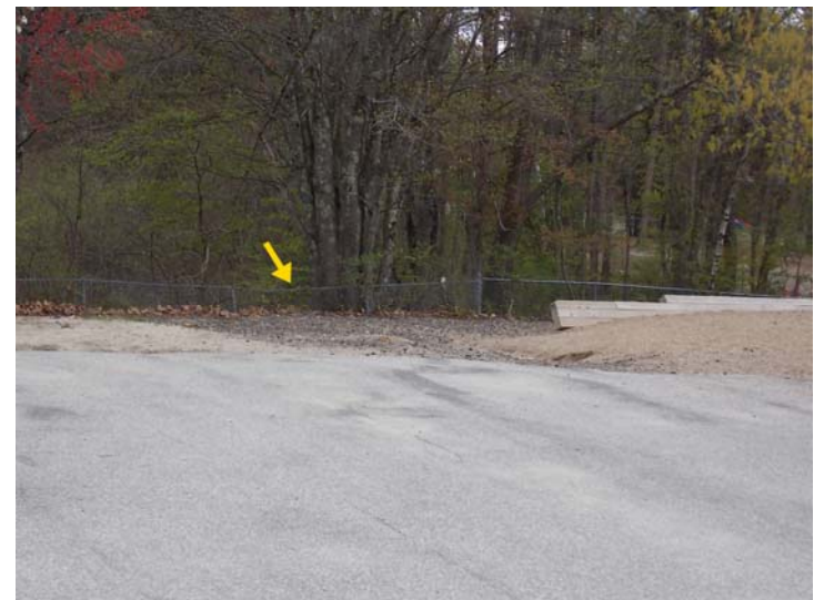
The height of the perimeter fence has been reduced by almost 50% due to the erosion at the playground.
