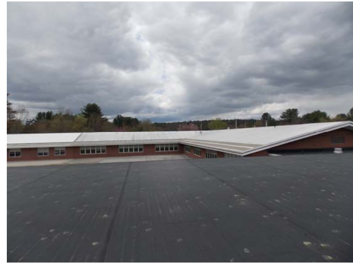
On the main building, the flat roof is covered with a rubber membrane and the pitched roof is covered with a PVC membrane.
