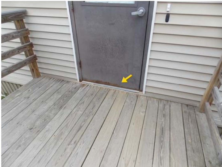
An exterior door on one of the portable buildings; note the rust at the bottom of the door.
