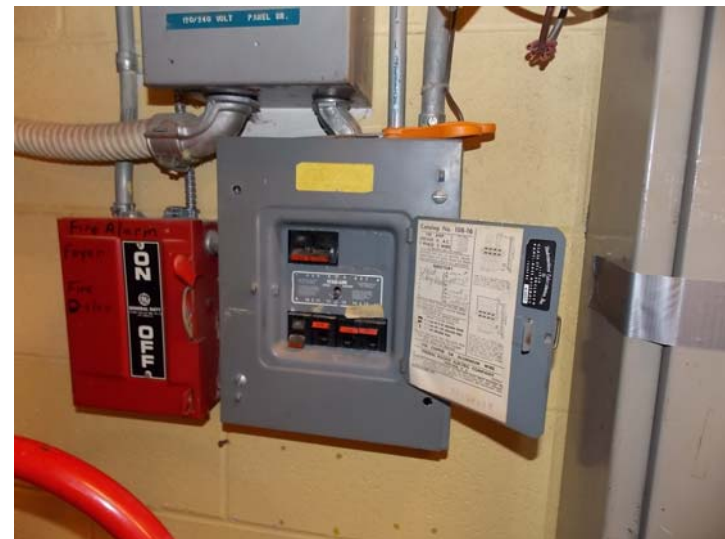
This FPE circuit breaker panel should be replaced in the near-term. These panels do not reliably react to electric overload conditions.
